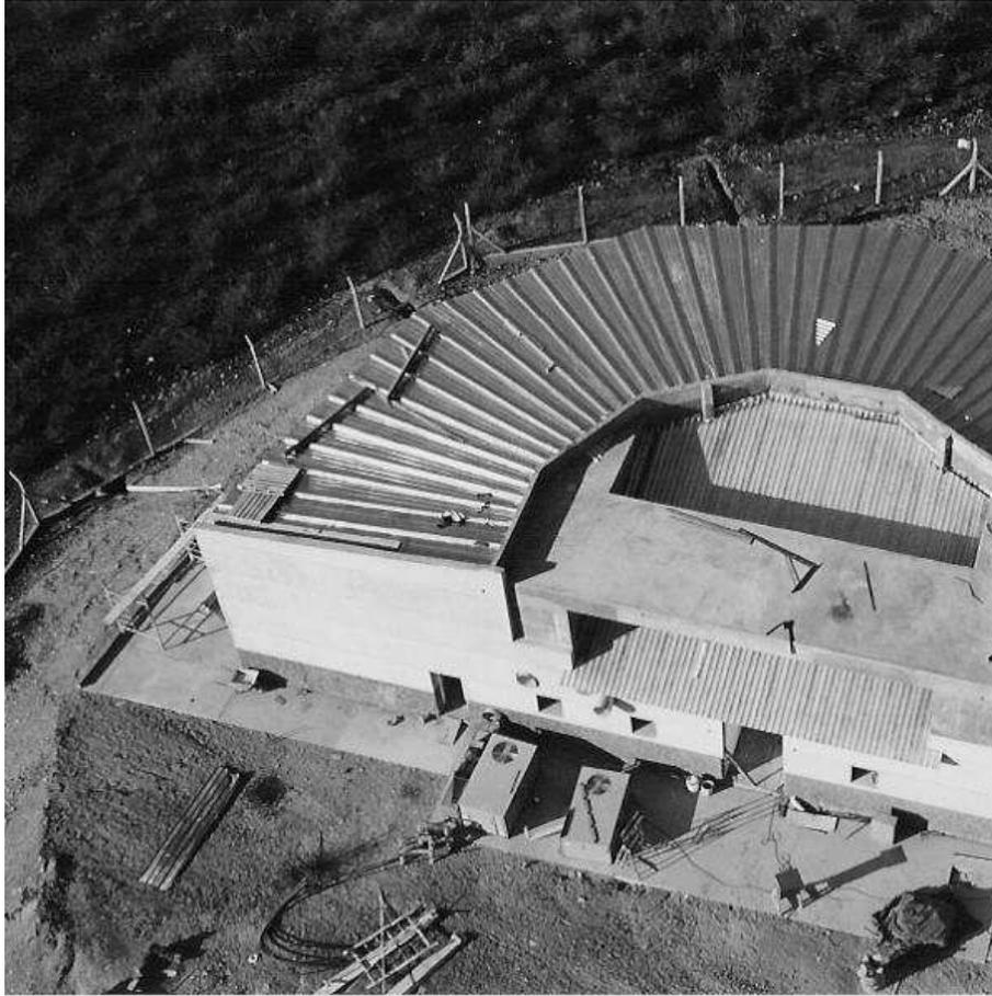
Figure 4: Top view of one of the four fluorescence detectors overlooking the surface array. It contains six telescopes , each with a field of view  $30^\circ \cdot 30^\circ$ , covering together  $180^\circ$  in azimuth (the half circle seen).
